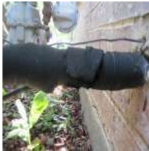
Deteriorate insulation
