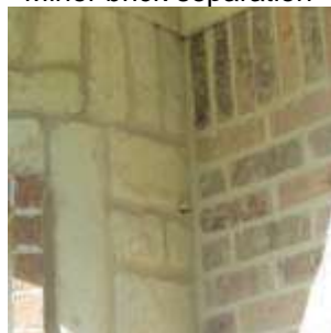
Deteriorated mortar
