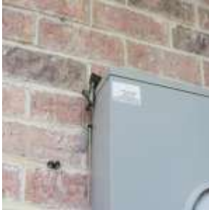
Improper grounding
