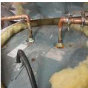
Galvanic corrosion
