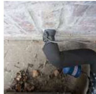
Deteriorate insulation
