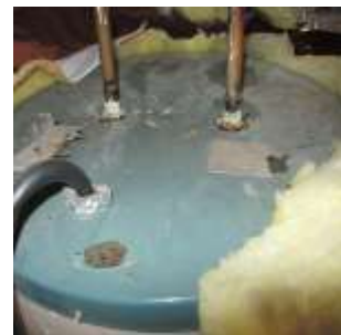
Galvanic corrosion
