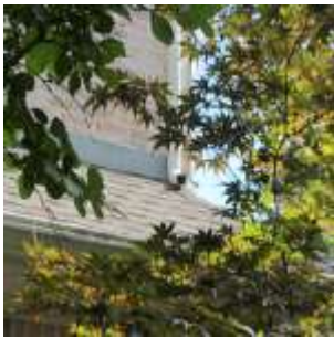
Downspout on upper roof
